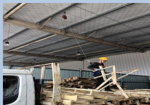
卸货点防坠落安全技改
